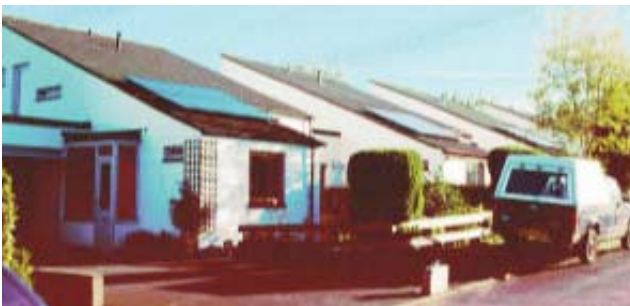
PV system installed on a residential property.
